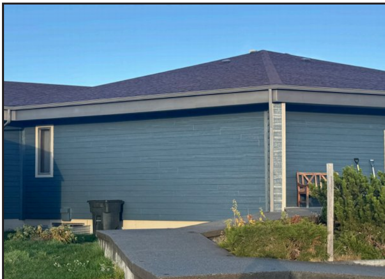
New siding and new color for the Bozeman church building “A nice blue, and a welcoming hue” Christ’s Church in Bozeman
